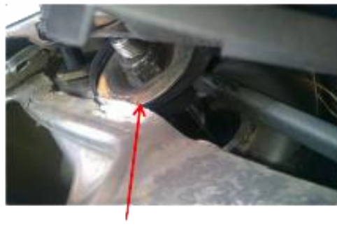
Low quality suspension bearing and insulator assembly Shock absorber shaft piercing through the body
